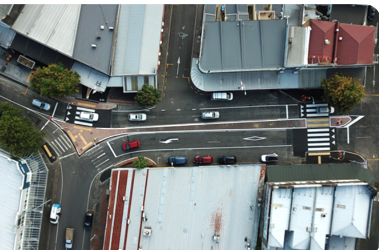
Fig. 1. Ponsonby Road-Pompallier Terrace site.
